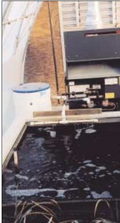
Heat exchange boiler influent received from the well pump.
