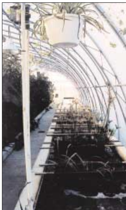
In the first bed, the leachate is aerated to encourage bacterial growth.
