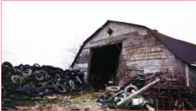
Abandoned tire dump near Hagersville, Ontario — site of the famous fire.
